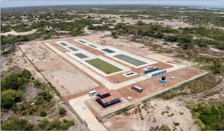
Kilinochchi Faecal Sludge Treatment Plant (25m 3 /day)
