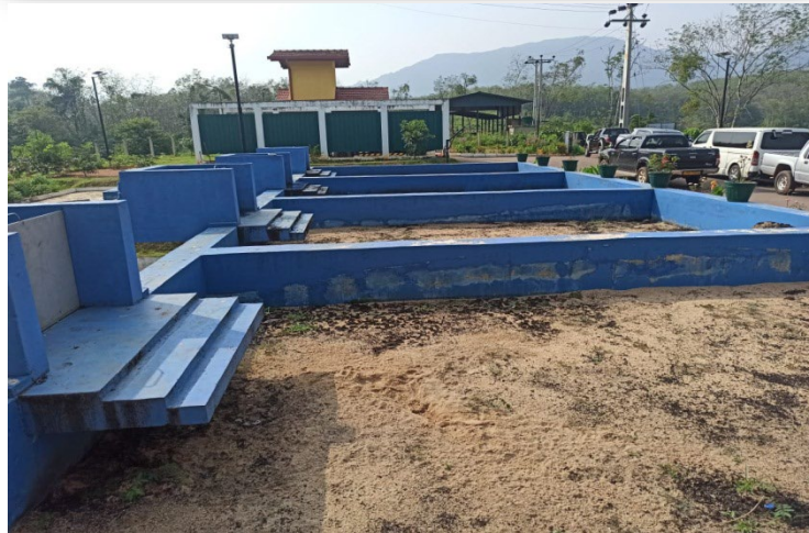
Weligepola Faecal Sludge Treatment Plant (25m 3 /Day)
