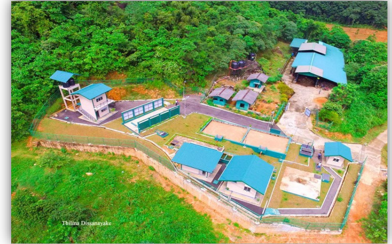
Ruwanwella Faecal Sludge Treatment Plant (25m 3 /Day)
