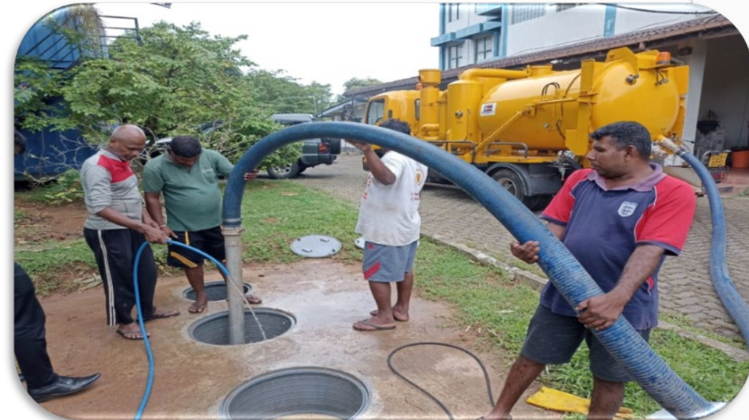
Desludging of the Johkasou system at the Ministry of Water Supply
