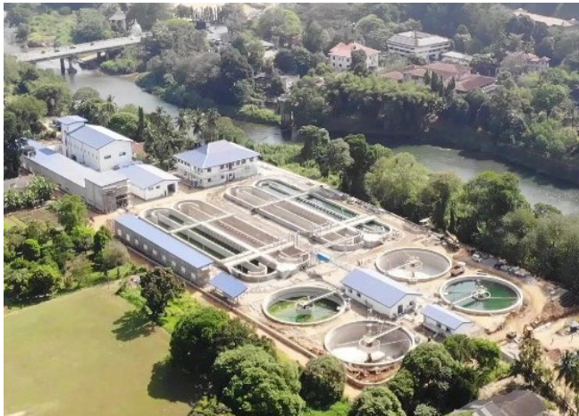
Kandy City WWMP- (Oxidation Ditch)
