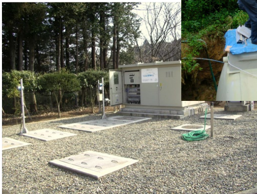
Upper concrete work
