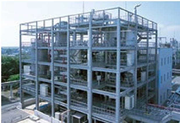
Sludge Treatment Plant
