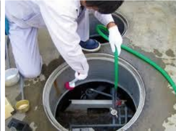
Clean inside tank
