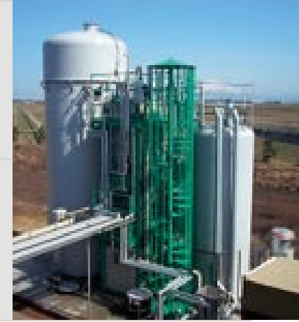
Anaerobic MBR
