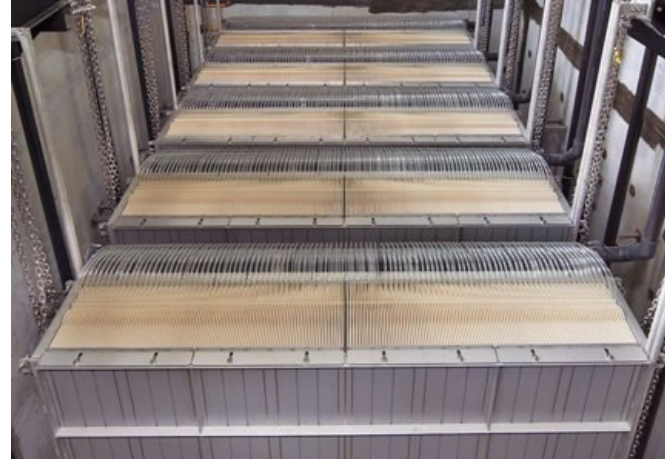
Submerged Membrane Unit (MBR)
