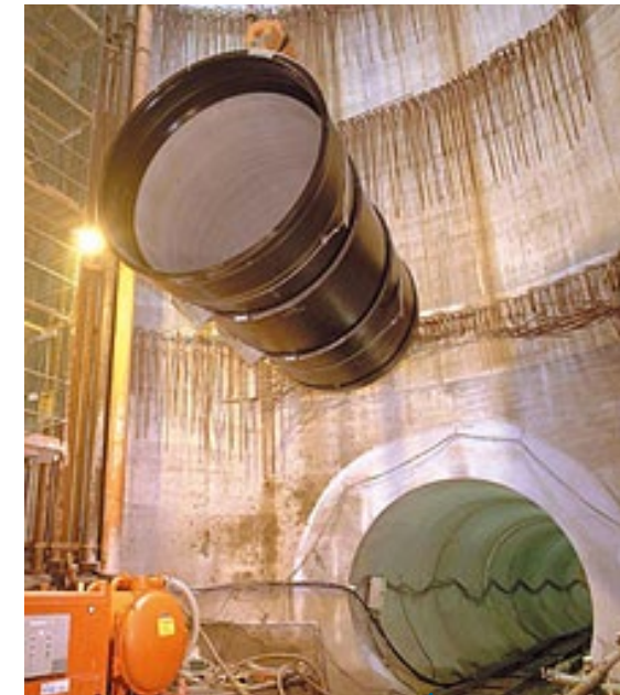
Ductile Iron Pipe
