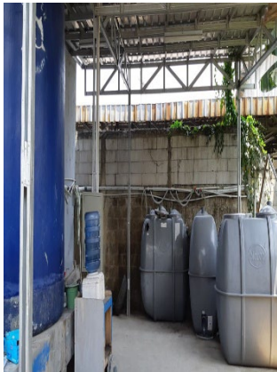
Leaking test in manufacture
