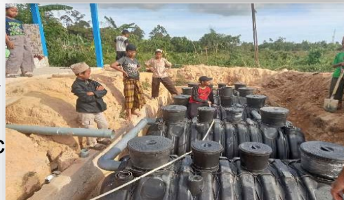
Prefabricated septic tank/biofilter tank
