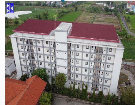
WWTP in Multistorey building, Surabaya City (PUPR)
