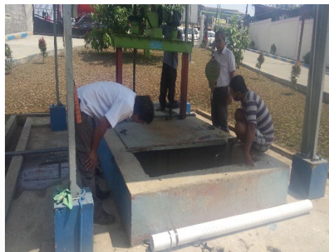
Gumuruh's centralized WWTP- Bandung City (water supply company)
