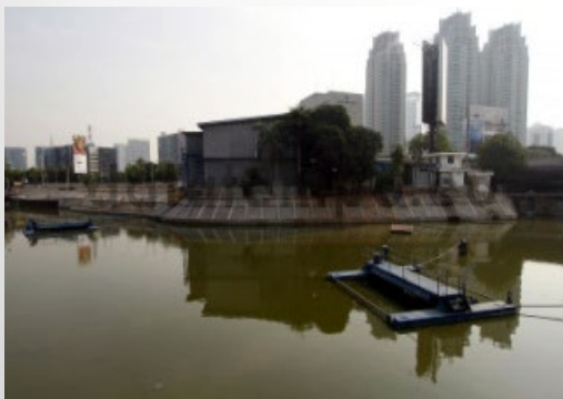
Setiabudi' centralized WWTP- Jakarta City (PD. PAL JAYA)
